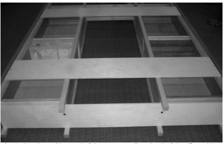
Attach the 2 vertical plywood ends to either end of the storage rails using 2 of the 1" machine screws supplied for each piece. (See image above)
